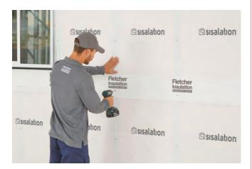
Recommended for temperate and cooler regions to help manage condensation. It allows vapour to escape the building, whilst helping stop vapour, water and wind from entering.
